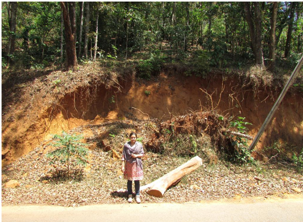
Photo – 16: View of debris slide in the west of Pudevettu (Slide Name – KAR/DK/48P09/2016/16) (Toposheet No – 48P/05).
