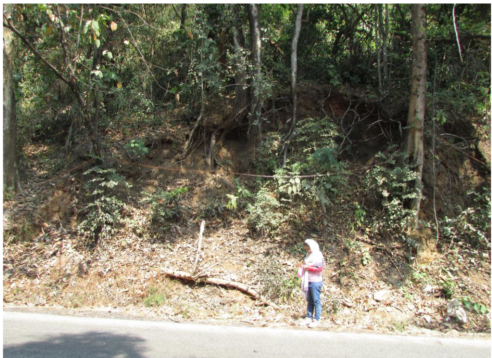
Photo – 14: View of debris slide along NH – 75 (formally known as NH – 48) in the east of Shradigadi (Slide Name – KAR/HAS/48P09/2016/05) (Toposheet No – 48P/09).
