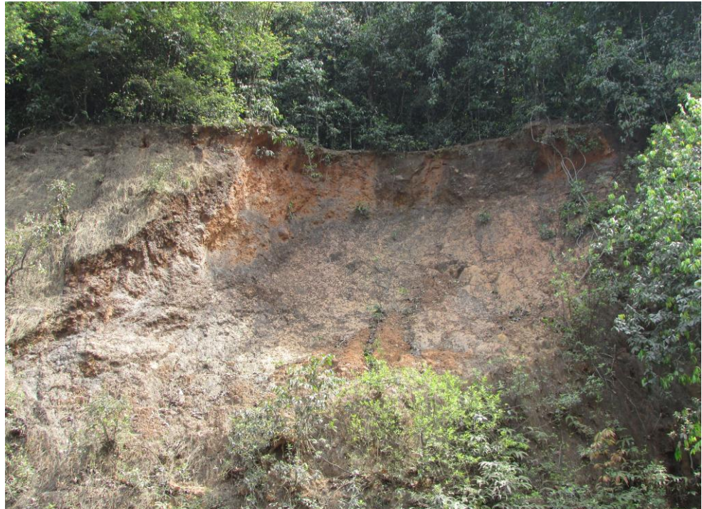
Photo – 13: View of debris slide along NH – 75 (formally known as NH – 48) in the east of Shradigadi (Slide Name – KAR/HAS/48P09/2016/04) (Toposheet No – 48P/09).
