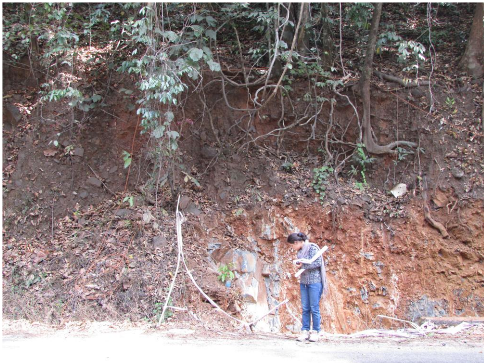
Photo – 12: View of debris slide along NH – 75 (formally known as NH – 48) in the east of Shradigadi (Slide Name – KAR/HAS/48P09/2016/03) (Toposheet No – 48P/09). The slide is almost wholly removed for maintenance of the NH.
