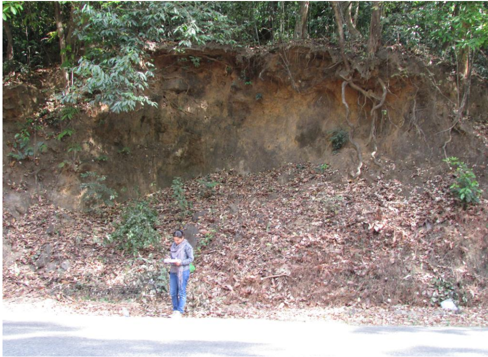
Photo – 11: View of debris slide along NH – 75 (formally known as NH – 48) in the east of Shradigadi (Slide Name – KAR/HAS/48P09/2016/01) (Toposheet No – 48P/09).
